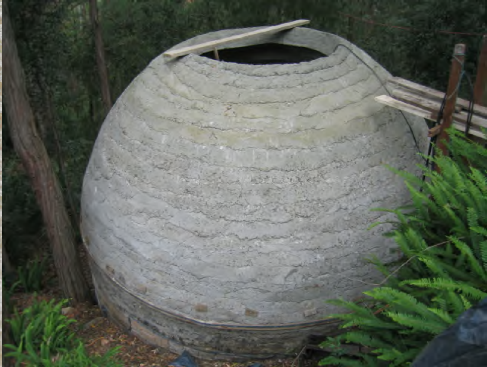
λ Papercrete dome extruded in Sydney, Australia
