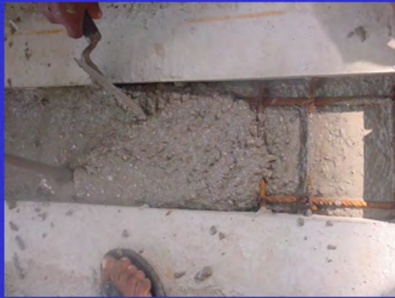
Geopolymer Concrete as fast setting material in joints of Precast Elements
