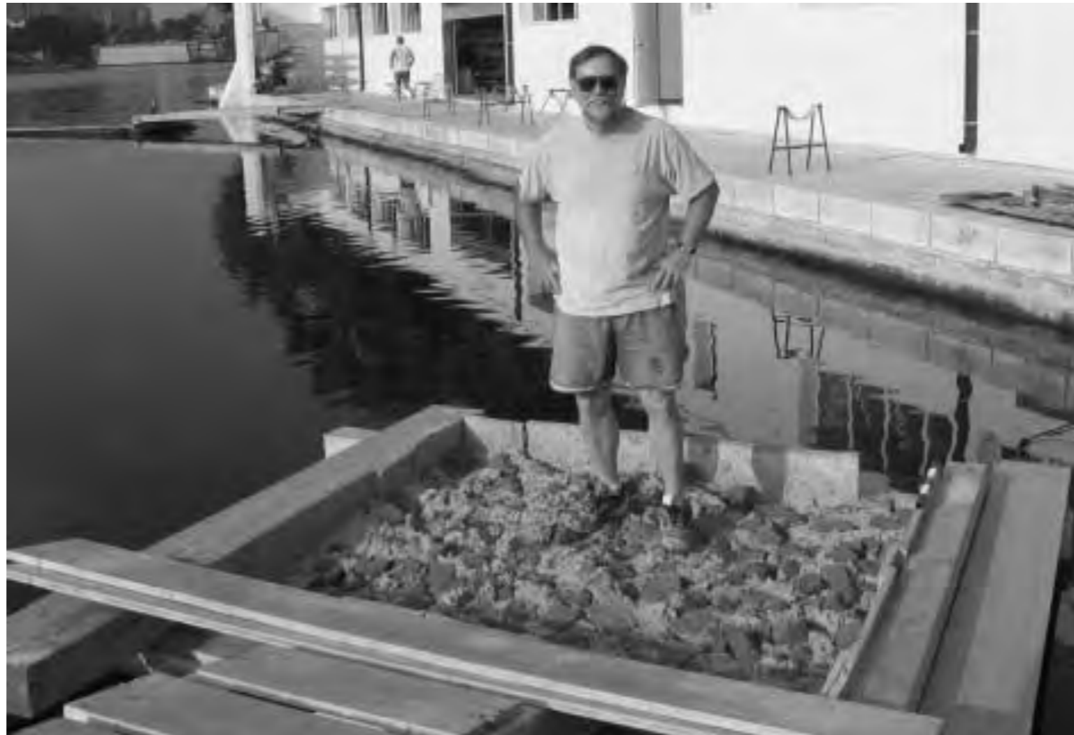
Figure 3. R. L. Hohlfelder stands on the concrete on the morning after the last mortar and aggregate had been placed in the form. (J. P. Oleson)
