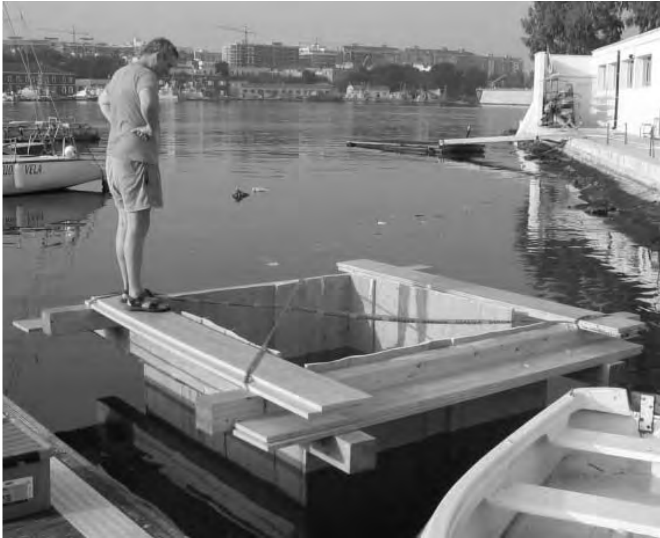
Figure 1. C. Brandon examines the completed form before filling. (R. L. Hohlfelder)
