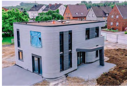
Peri 3D construction, Germany
