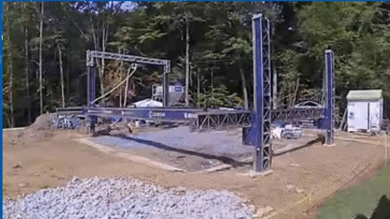
3D-Printed House Construction Time-Lapse
