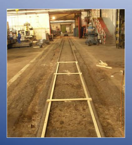
Fixing an old industrial floor close to the rails in steel producing factory. The deepness of floor gaps were from 2 mm to 20 cm.
