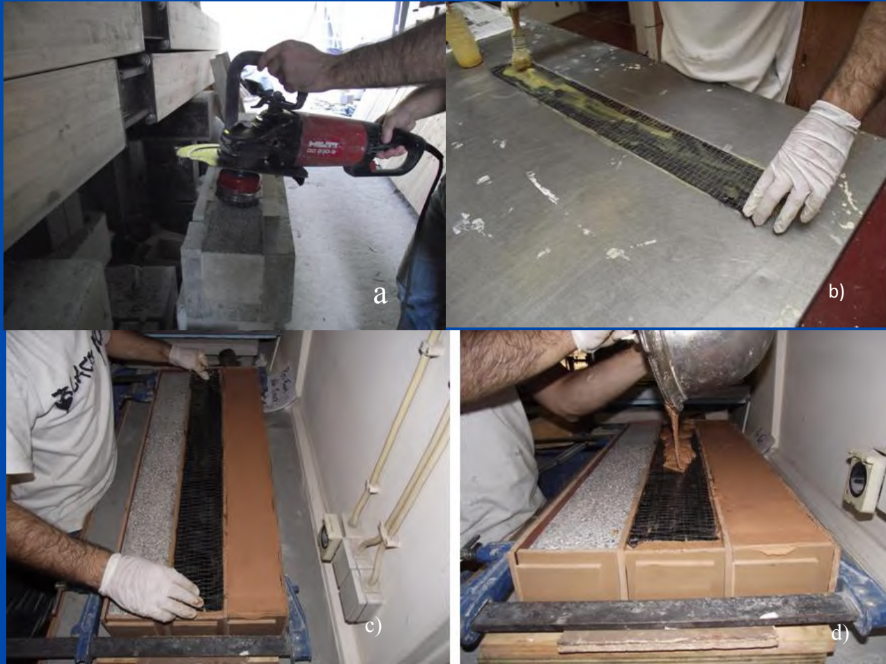
Figure 5 – OPC concrete beams preparation: a) surface roughening ; b) CFRP sheets impregnation; c) Placing the CFRP sheet over the geopolymeric mortar; d)Applying a second layer of geopolymeric mortar
