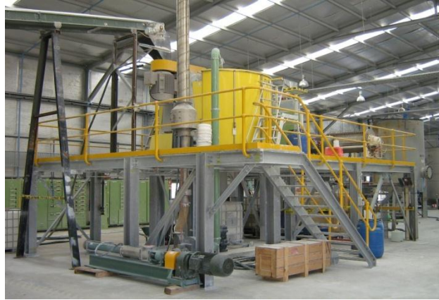
Full scale mixing and granulation
