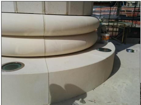
These are the outter column base. It is segmented in 10, and each segment is a set of two parts, a "M" shaped and a "L" shaped part.
