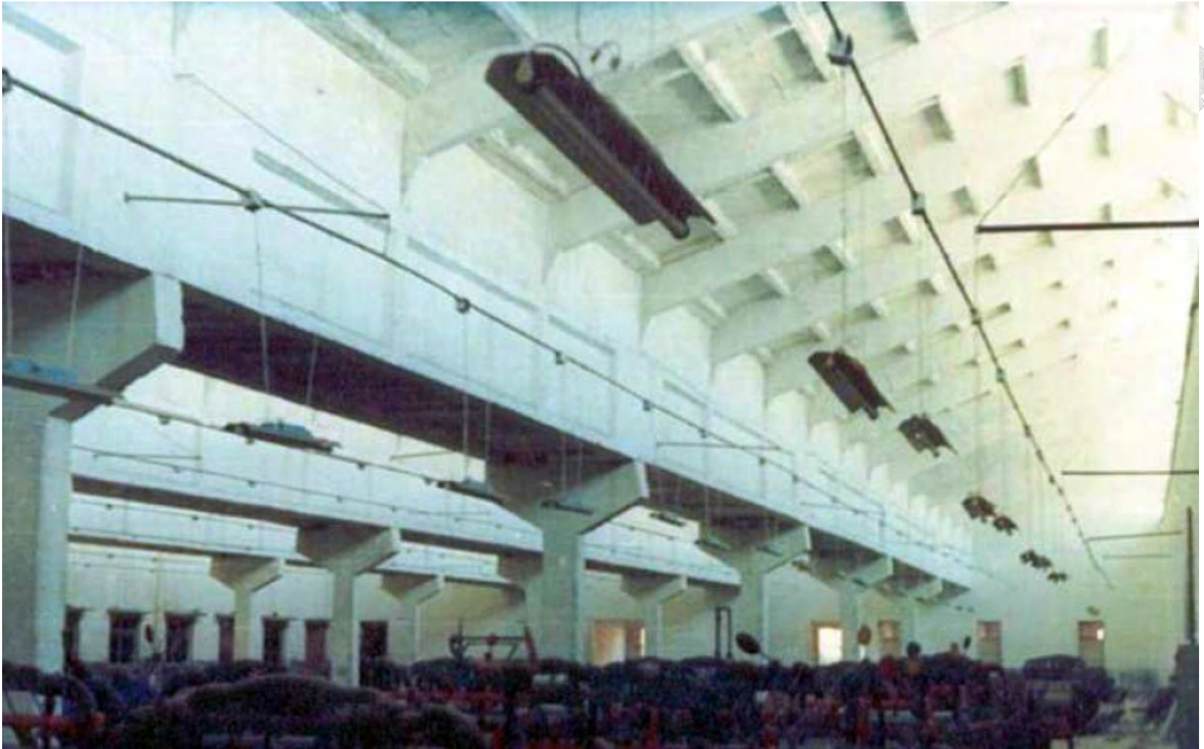
Beams & columns of a workshop
