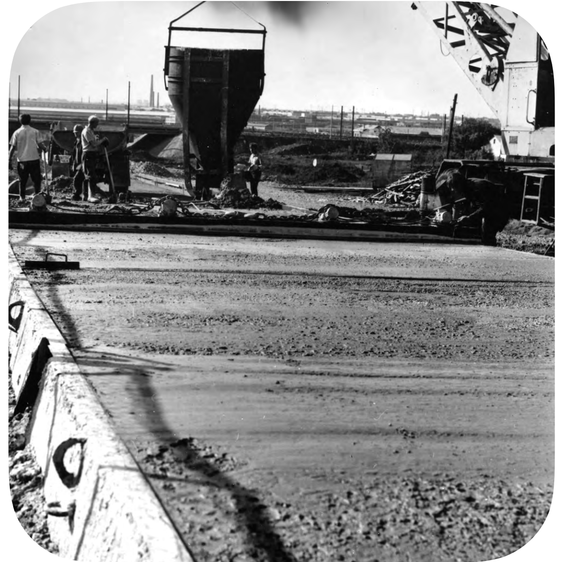
Process of road construction with alkali-activated concrete, length 6 km, to the quarry of mountain Magnitnaya. Magnitogorsk, Russia, Ural, 1984, inspection visit in 1999.
