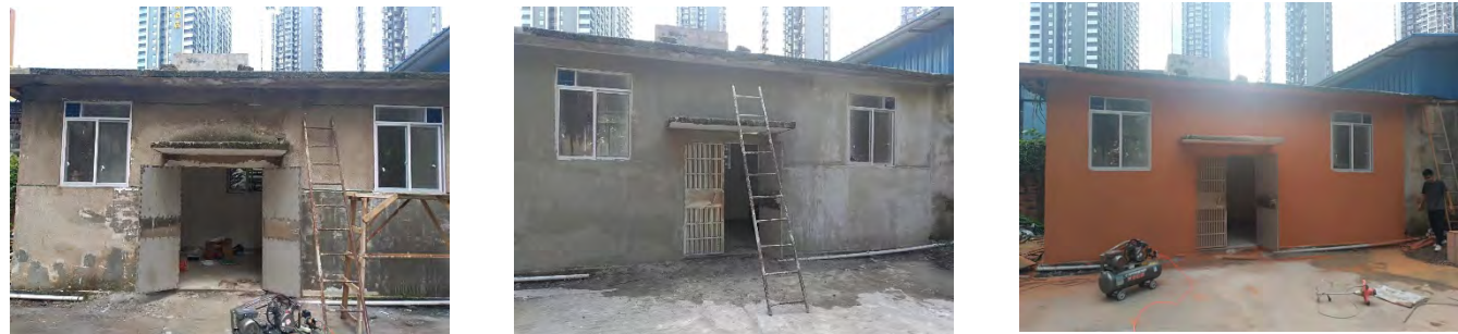
Geopolymer coating used in emergency repair engineering Nanning city, China, 2019
