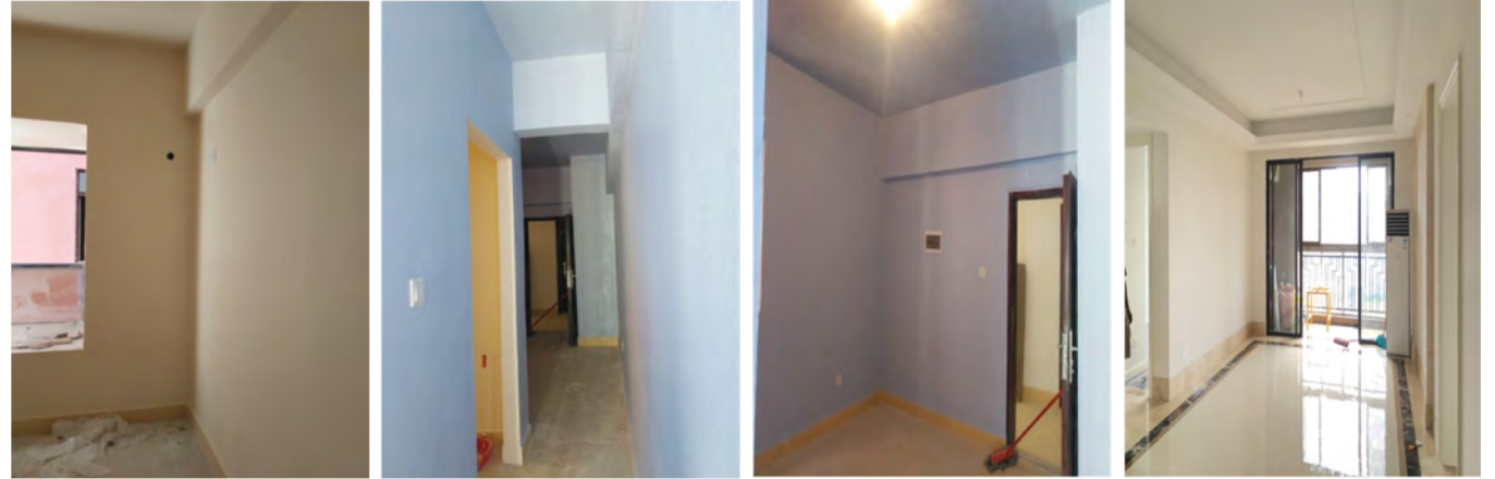
Application of geopolymer coating in engineering Nanning city, China, 2018
