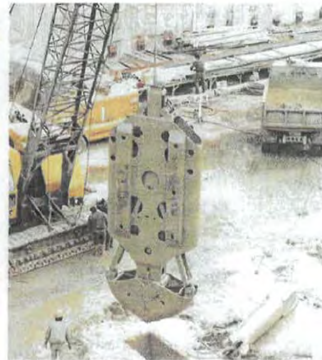
MECHANICAL CABLE BUCKET GRAB
