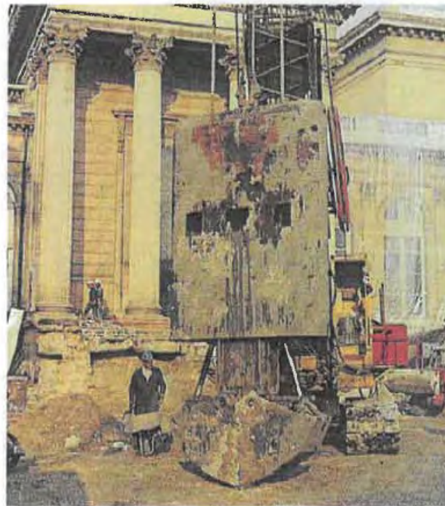
HYDRAULIC CABLE BUCKET GRAB
