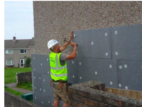
Better insulation and heating
