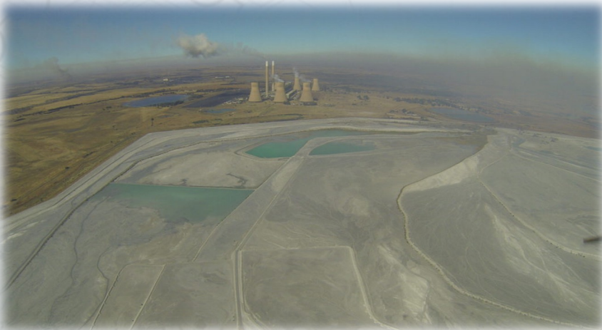
Ash dam: Mpumalanga, South Africa
