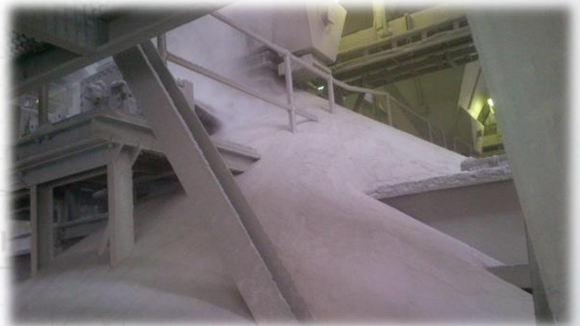
Ash disposal problems: Lethabo Powerstation
