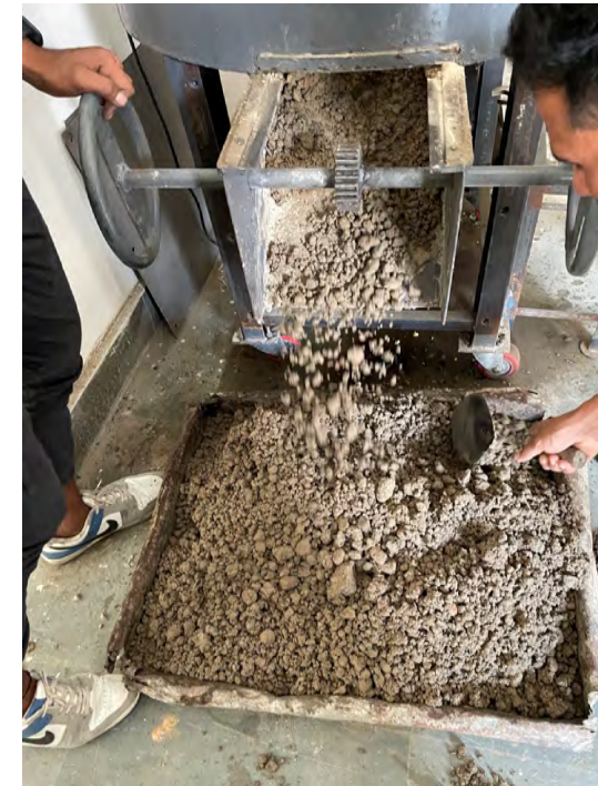
Treated mix for base layer application
