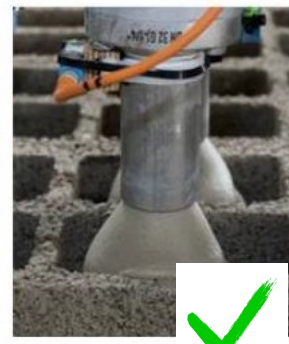
Filling up of cavities or under the roof → Walls up to 3 meters !
