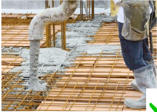
To reduce amount of concrete
