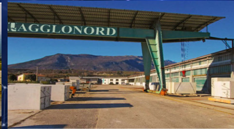
Slabs production plant Rivoli Veronese / Italy
