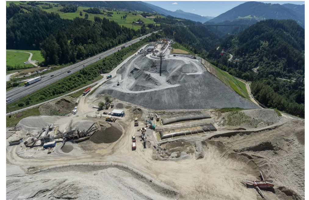
[Processing facility and deponie Brenner Base tunnel, 2022]
