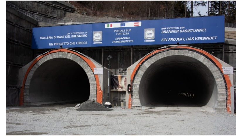
[Brenner Base tunnel]
